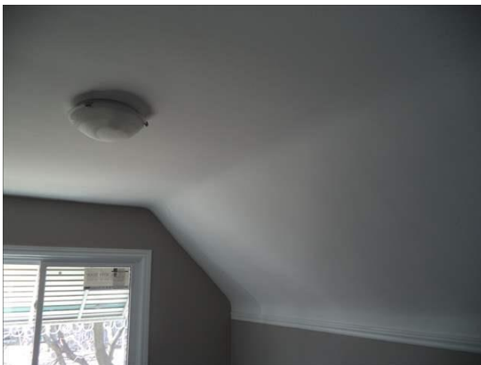
Typical image - above rear bedroom
